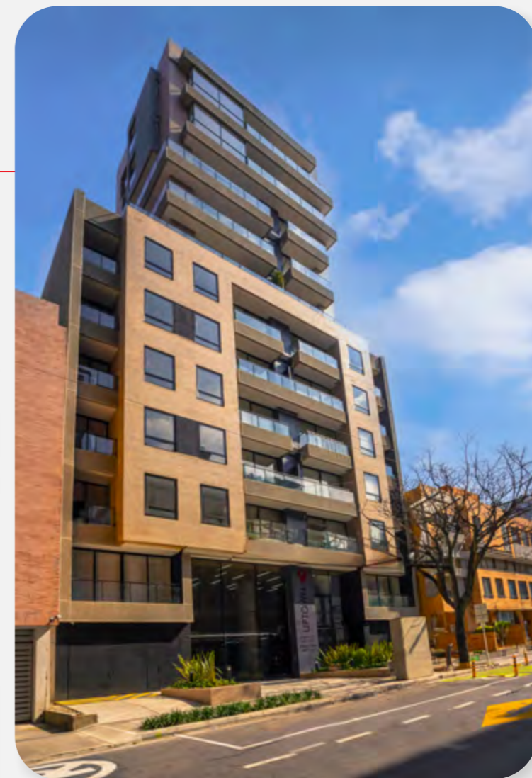
Uptown 127 / Mayor a VIS Dor Construcciones S.A.S. Bogotá
