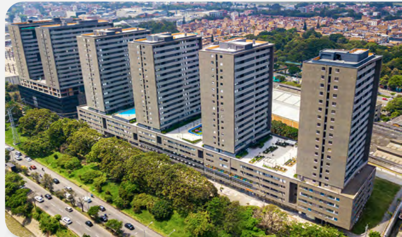
Urbanity / Mayor a VIS Constructora Capital Medellín S.A.S Medellín
